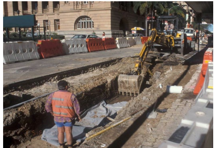
Figure 1. Installation of street tree pits
